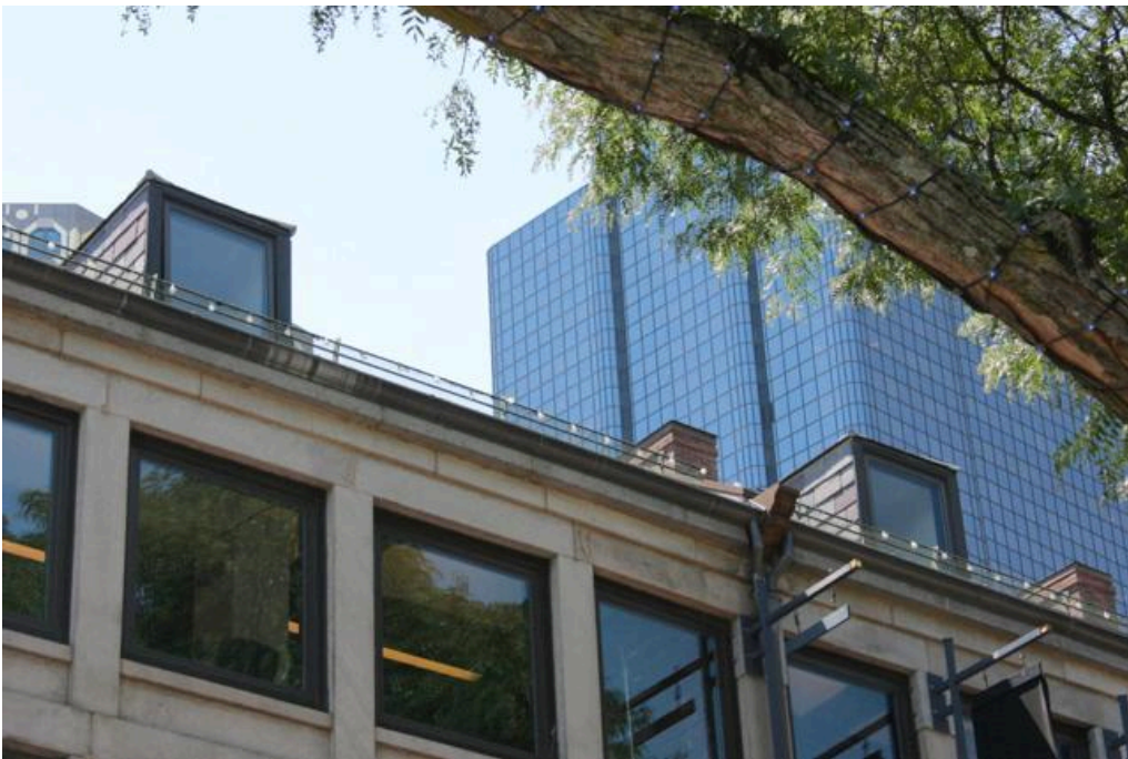
Figure 9. Façade (north elevation): Detail of roof edge.
