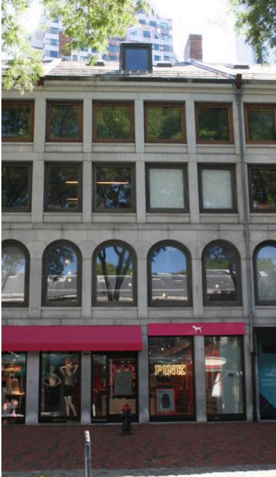
Figure 6. Façade (north elevation): Typical four-bay building unit.
