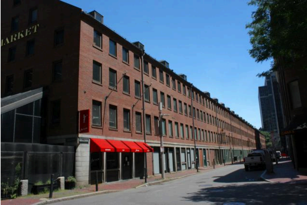
Figure 16. South elevation, looking east.
