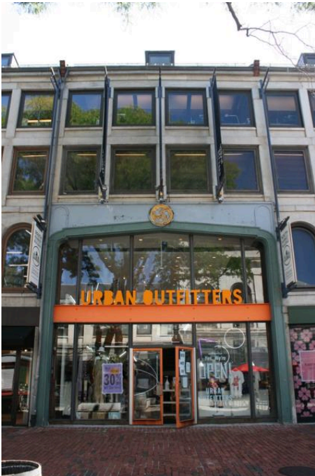
Figure 11. Façade (north elevation): Detail of storefront with two-story arched frame.
