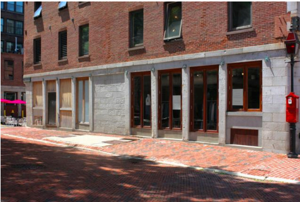
Figure 13. East elevation: Detail of first floor.
