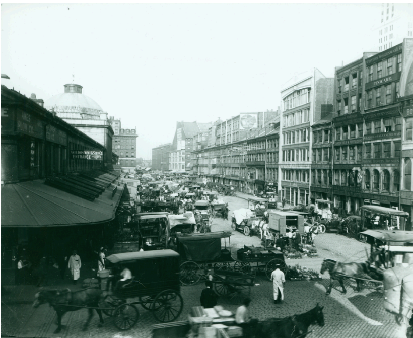
Figure 22. South Market St., ca. 1915-1925. View east from Merchants Row, showing Faneuil Hall Market at left, and fifth- and sixth-story additions on South Market buildings at right, with Custom House behind.
