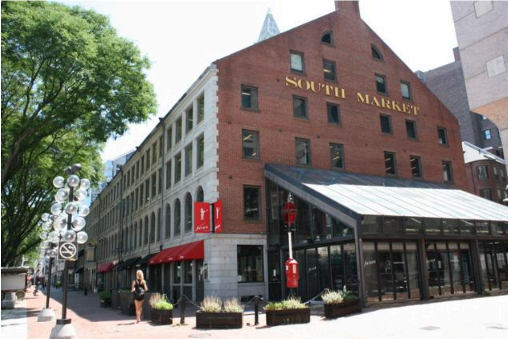
Figure 2. Façade (north) and west elevations, looking southeast.
