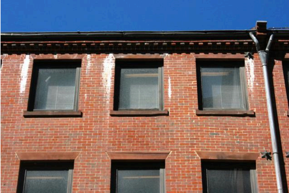
Figure 18. South elevation: Detail of windows and roof edge.
