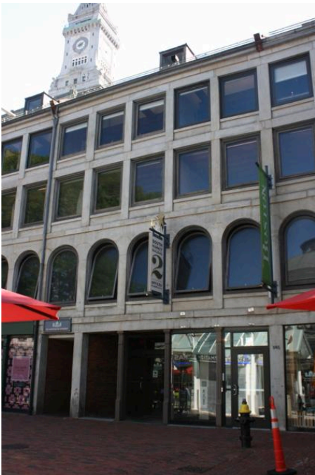
Figure 7. Façade (north elevation): Five-bay unit in center of block includes Entrance 2 to upper levels of the block, and a public passage.
